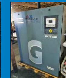
20-HP Atlas GA15-VSD Air Compressor
