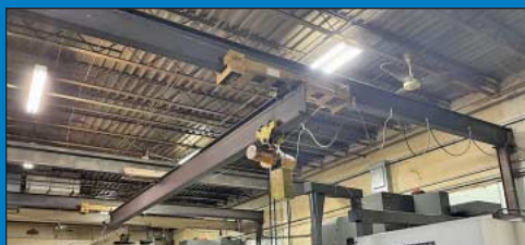
(9) Bridge and Monorail Crane Units with Hoists
